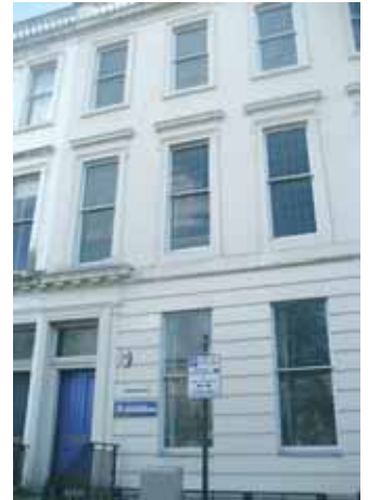
Above: The new premises in Newton Terrace, a short distance from the old practice
